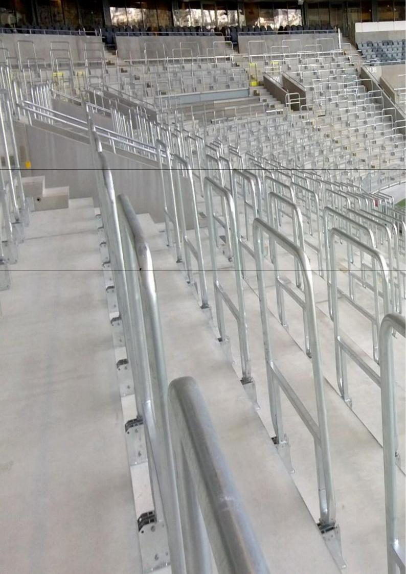
Installation of **fast – latch** at the Tele2 Arena – Stockholm – Sweden. Shown here in standing mode the 'combination area' can be very quickly and efficiently converted to seating mode shown on the adjacent page.
