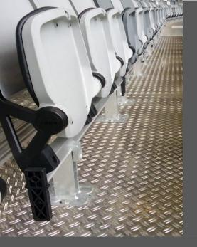
This image shows the demountable terrace closure for the lower terrace access apertures used when the arena is in concert mode - shown here in sport mode 3 seat units are floor (tread) mounted to the de-mountable terrace sections – when taken out the seat units can be handled and stored in our standard aluminium stillages.
