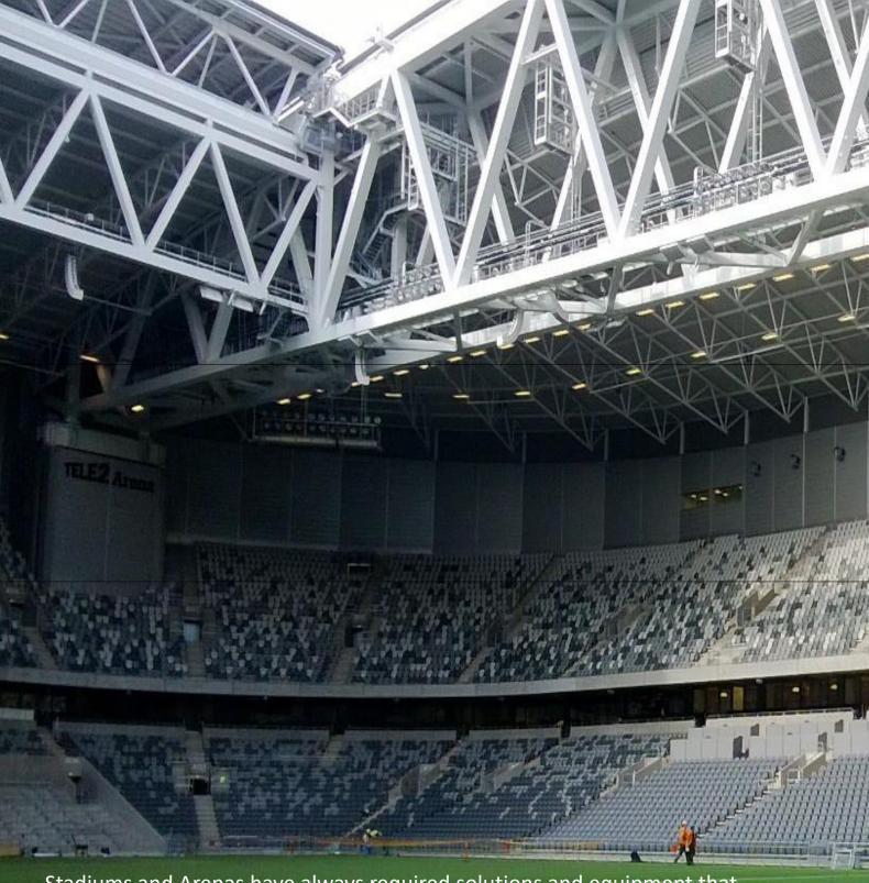
Stadiums and Arenas have always required solutions and equipment that facilitate the adaptation of a building to different modes of operation. Telescopic grandstands are used to help 'flex' space - to bring seating closer to and further away from the field of play - to adapt sight lines to meet the requirements of different sports or events.
