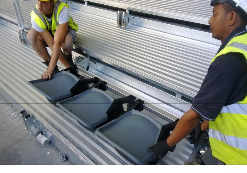
**fast** – **latch** mechanisms are available with a secondary fold-down function so that they can be used on telescopic units – at the Tele2 Arena the telescopic unit is also used in seating and standing mode – in either seating or crush-rail mode the telescopic can be closed without removing the rails or seats.
