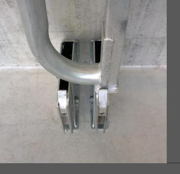
When in standing mode crush rails are intermittent so that the standing crowd has free movement on the terrace – the 'overhanging' design of the crush rail ensures that the adjacent mechanism is made safe and does not cause a trip hazard.
