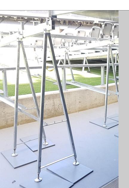
Elevated on our 'A frame' substructure; multi deck is the simplest and fastest build system on the market! Seating is arranged on 'ladder beam' risers which serve as a seating rail and transverse structural brace, whilst also supporting the front and rear of each deck. The system reduces install time and labour, allowing seats to be compactly stored into stackable stillages. See our time lapse build video.
